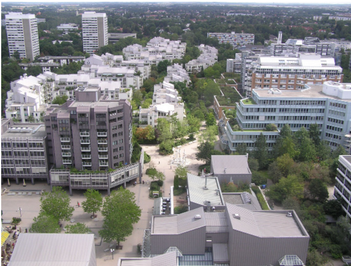
Figure 38: Arabella Park TOD on the U4 U-Bahn line, Munich.
