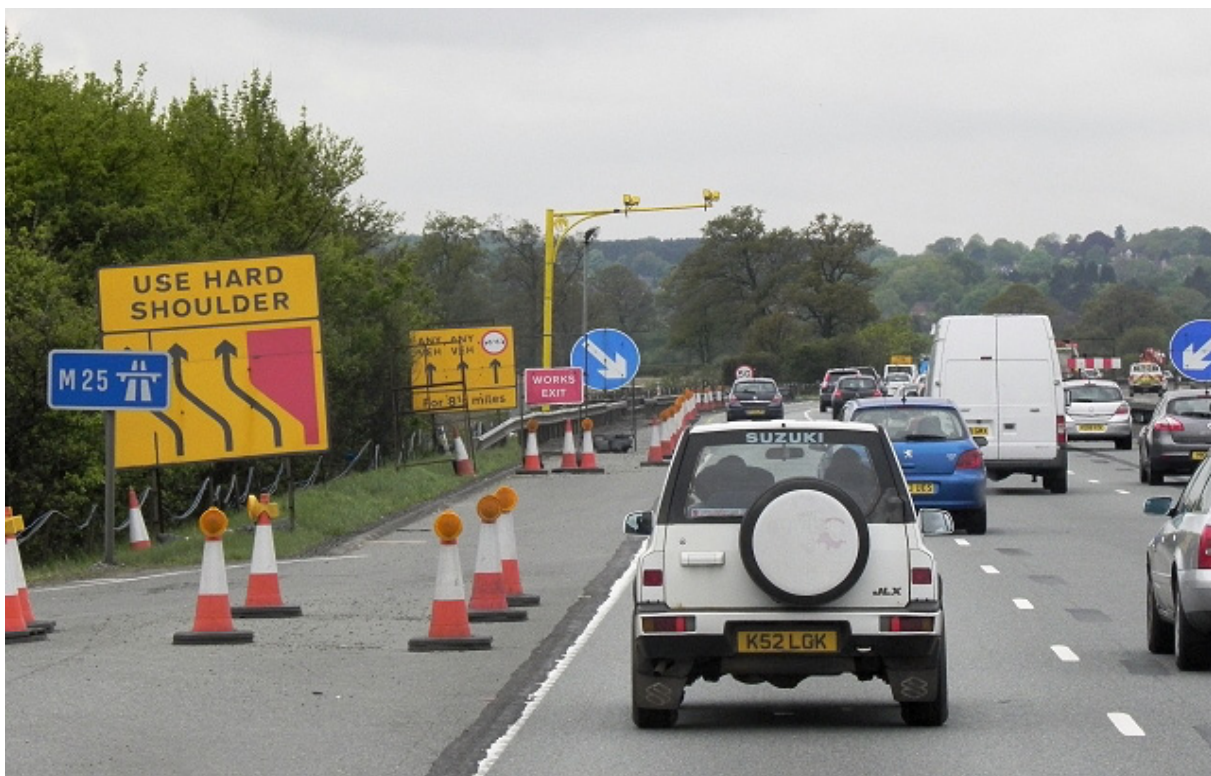
Plate 8: M25 Roadworks, England
