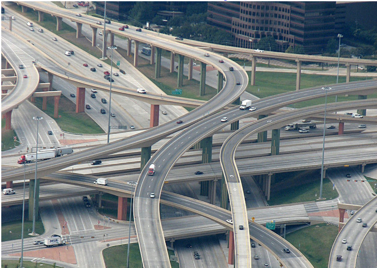
Plate 7: High-Five interchange, Dallas, USA
