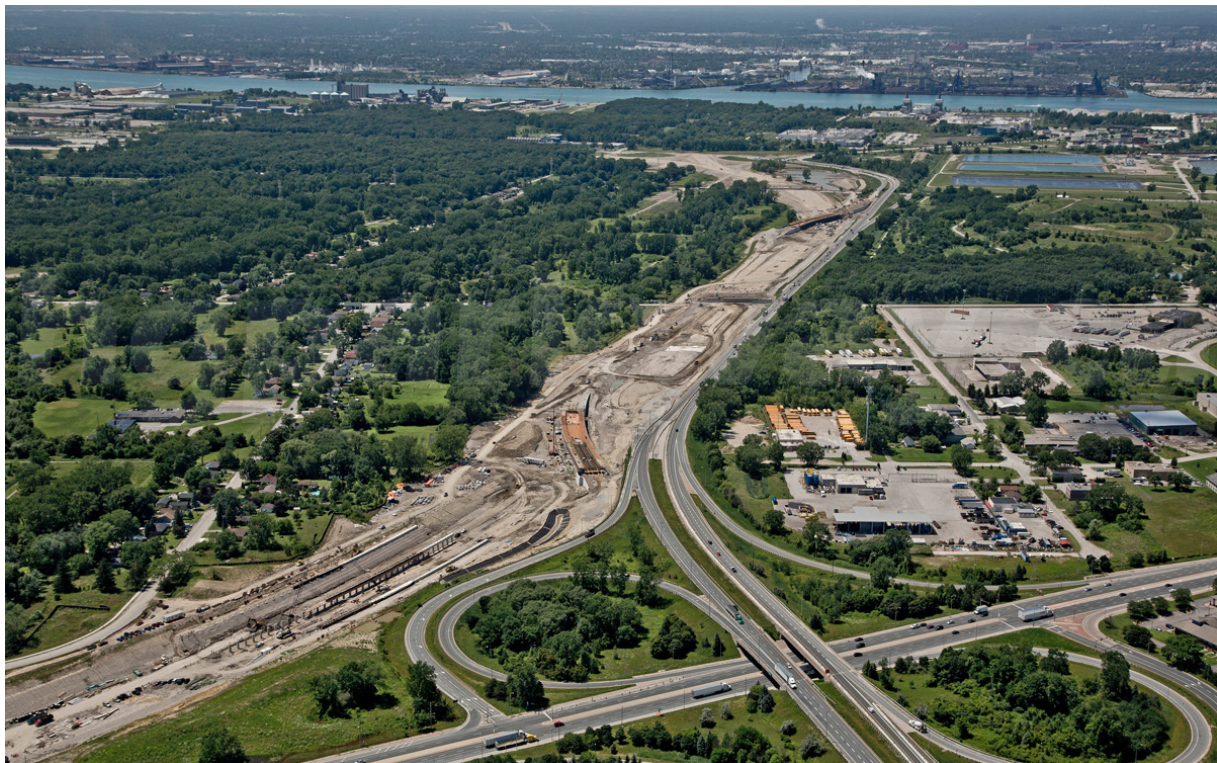
Plate 10: Ontario highway 401, Canada
