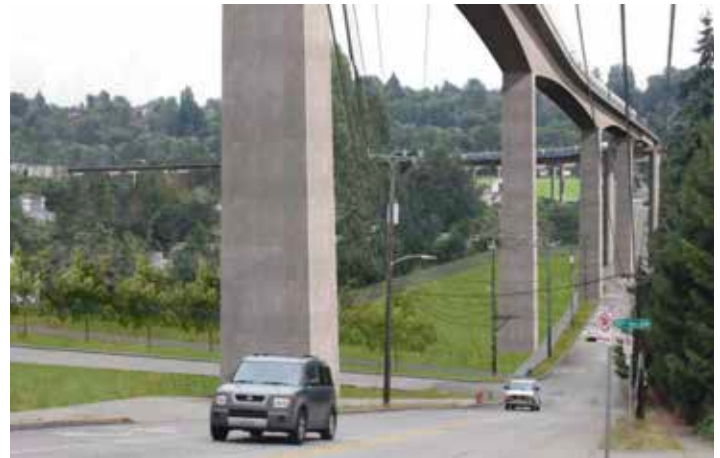
Figure 2: SW Genesee St. with a rendering of the proposed light rail guideways (Source: Sound Transit WSLE DEIS)
