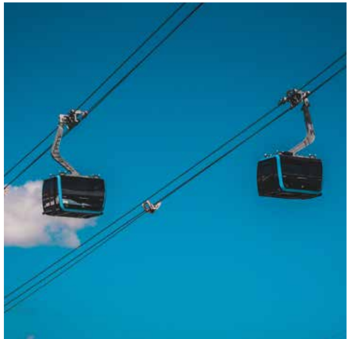
Photo credit: Christian Meyer, Two crossing cabins of the cable car from Trockener Steg to Kleines Matterhorn above Zermatt in the Swiss Alps, LEITNER ropeways, Trockener Steg, Zermatt, Switzerland, 2022. https://unsplash.com/photos/a-group-of-cars-on-a-cable-HM8HhmYP4N8
